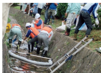
Exercise of piling up sandbags along a conduit (Shiga Prefecture)
